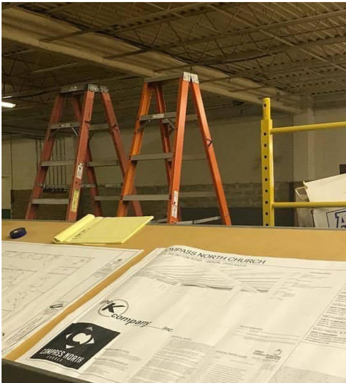
Construction #1: Plans are laid out as work begins.
